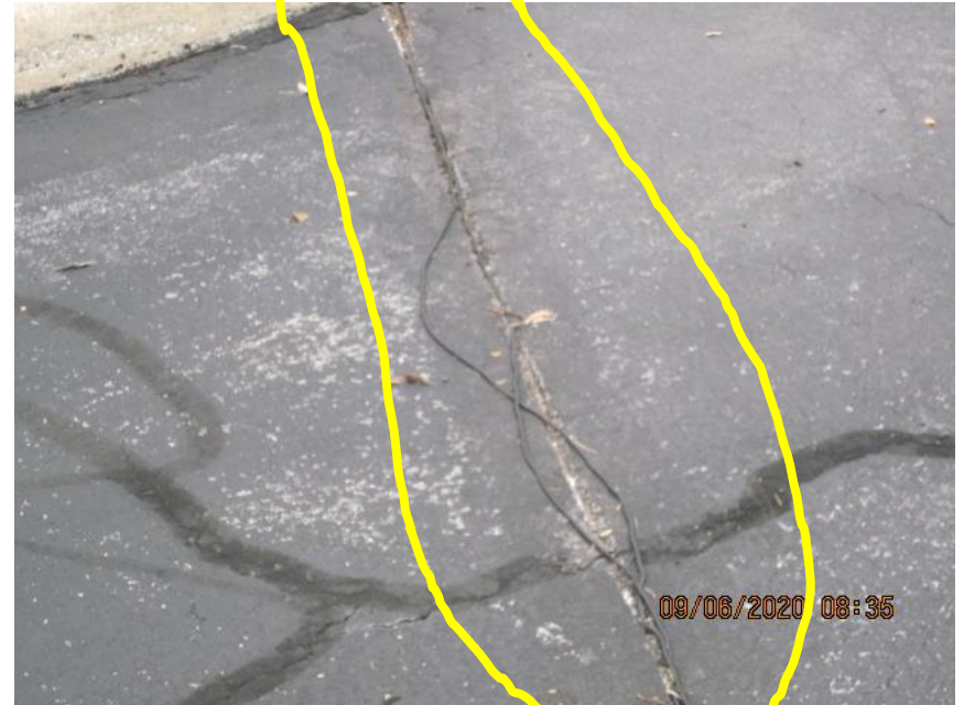
Entrance interisland low voltage Wiring [removed]
