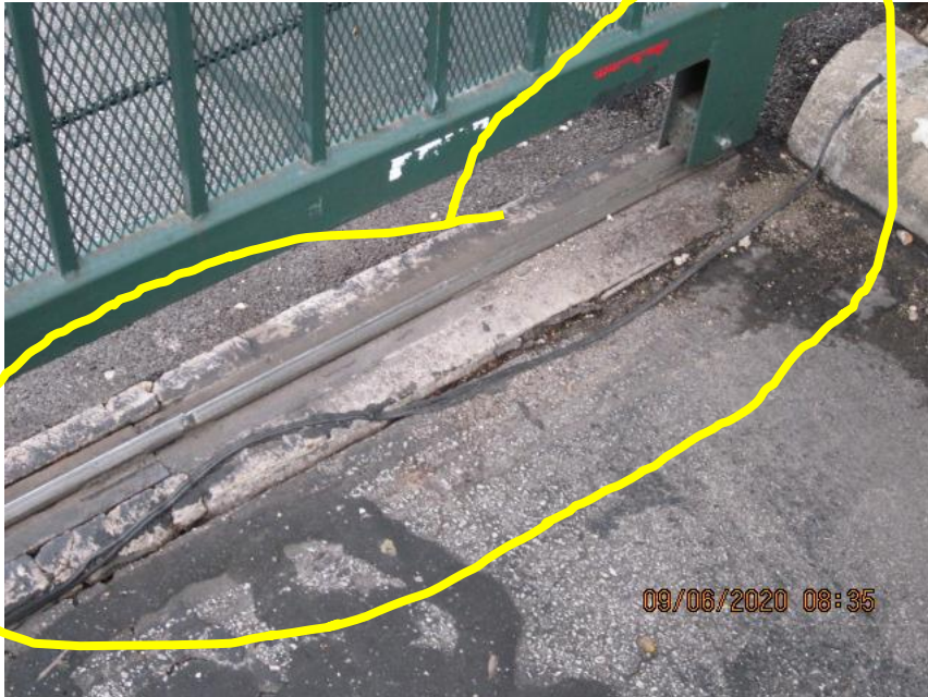
Entrance low voltage wiring: Unsecured along entrance & exit gate tracks
